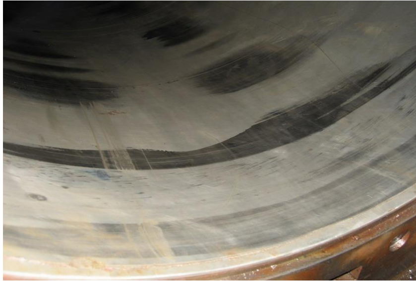
Figure 9.1.2 Melting of Tube Afterward Bearing due to Poor Shafting Alignment
